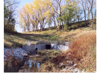
Flared outlet (wing wall)
