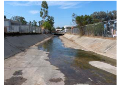
Trapezoidal concrete channel
