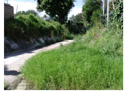
Low-flow concrete channel with natural sides
