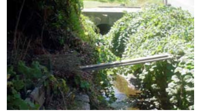
Circular culvert and natural-lined channel
