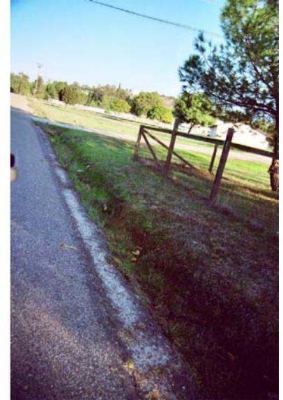
Brow ditch adjacent to roadway
