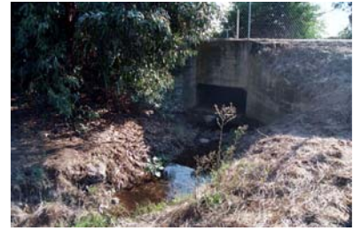
Rectangular culvert and soft bottom channel
