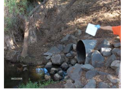
Corrugated metal pipe outfall
