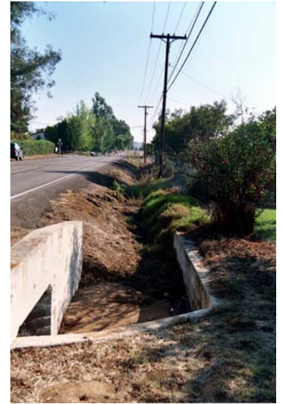
Box culvert and natural-lined ditch
