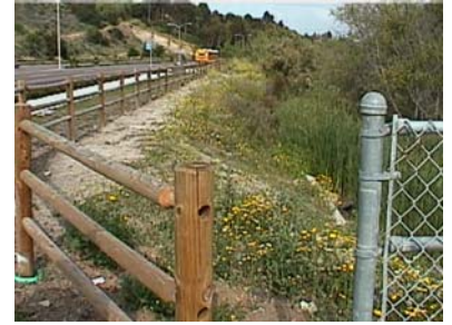
Earthen storm channel
