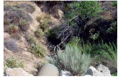
Pipe outlet into earthen channel
