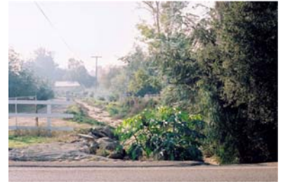
Earthen channel with riprap slopes near culvert
