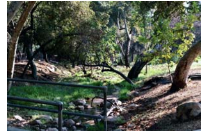
Upstream of inlet along natural-lined channel
