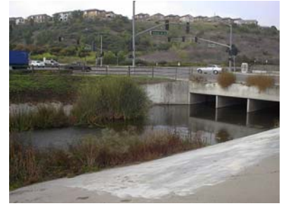
Concrete-lined inlet to box culvert
