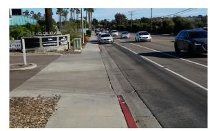
FIGURE 4.7.8. MISSING TRUNCATED DOMES ON VIA DE LA VALLE
