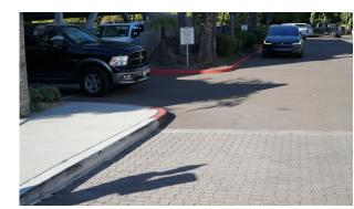
FIGURE 4.7.9. LOW-VISIBILITY CROSSWALK AND MISSING CURB CUTS IN PARKING LOT OFF VIA DE LA VALLE
