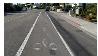
FIGURE 4.7.12. UNPROTECTED BIKE LANE WITH FADED MARK-INGS ALONG VIA DE LA VALLE
