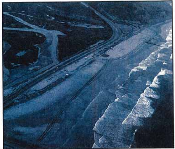
Figure 5.6. Aerial view of the Torrey Pines beach fill project (from Seymour, et.al., 2005).
