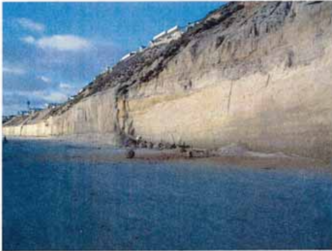
Note: Bluff Failure Stopped at Seawall
