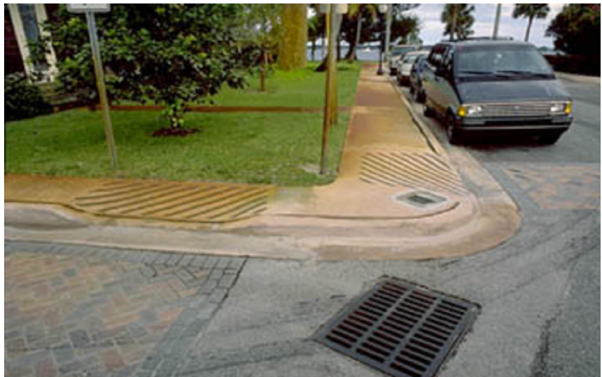
Photo Courtesy of: http://www.pedbikeimages.org/ Peter Lagerwey
