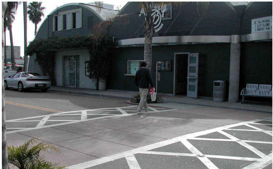
This raised pedestrian crosswalk is located on Cedros, just south of Lomas Santa
