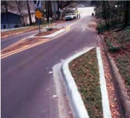
This chicane has been built away from the existing curb to maintain drainage. As can be seen from the photo, debris has a tendency to collect between the device and the curb. Photo Courtesy of: www.pedbikeimages.org / Dan Burden
