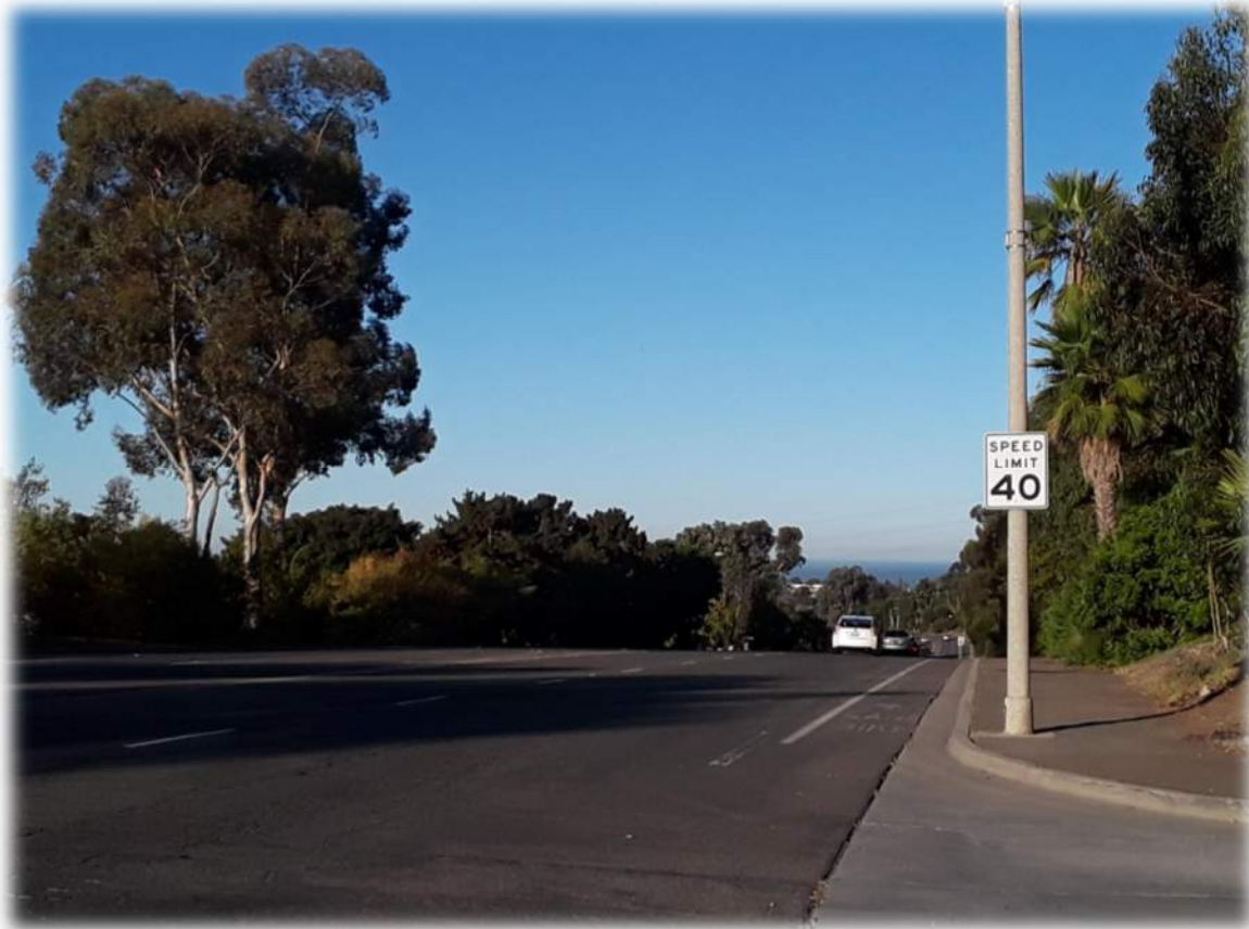
Looking Westbound on Lomas Santa Fe east of Granados Avenue
