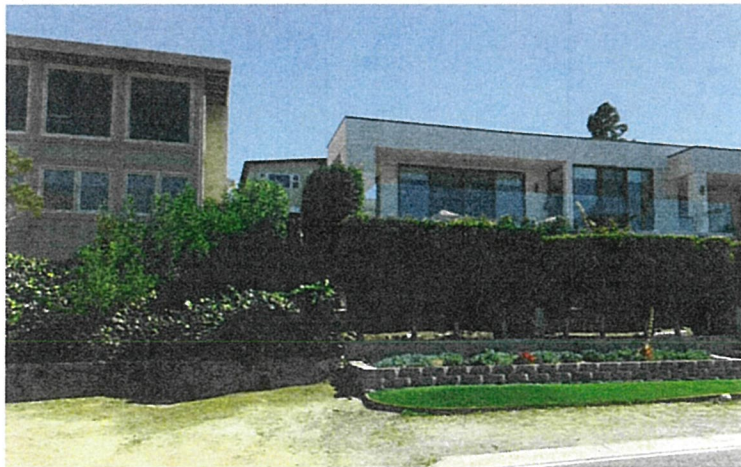
3. VIEW TO SOUTHEAST FROM FRONT OF HOUSE
