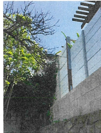
6. VIEW TO SOUTH EAST FROM REAR YARD
